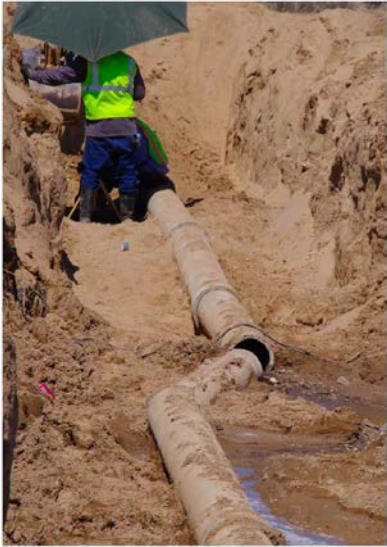
Damage to buried pips in 2019 M7.1 Ridgecrest event
